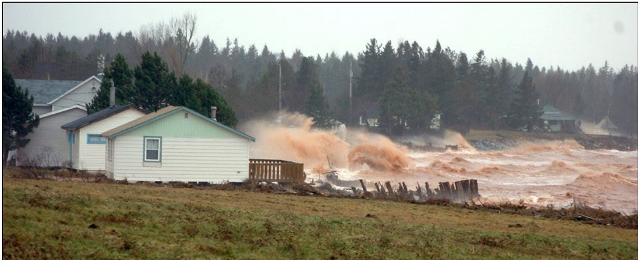
Figure 10. A photo from the Amherst Daily News which depicts waves impacting a portion of coastline west of River Phillip along the Northumberland Strait on December 21 st of 2010.
